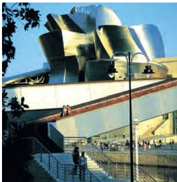
Lávka u Muzea Guggenheim / Footbridge at the Guggenheim Museum, Bilbao
