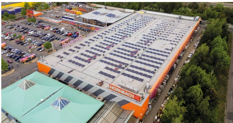
Foto: Archiv S-Power Business Solutions
